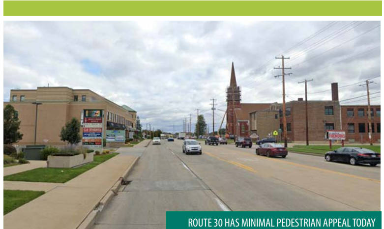
ROUTE 30 HAS MINIMAL PEDESTRIAN APPEAL TODAY HART ST. & ROUTE 30 INTERSECTION NEEDS TO BE SAFER
