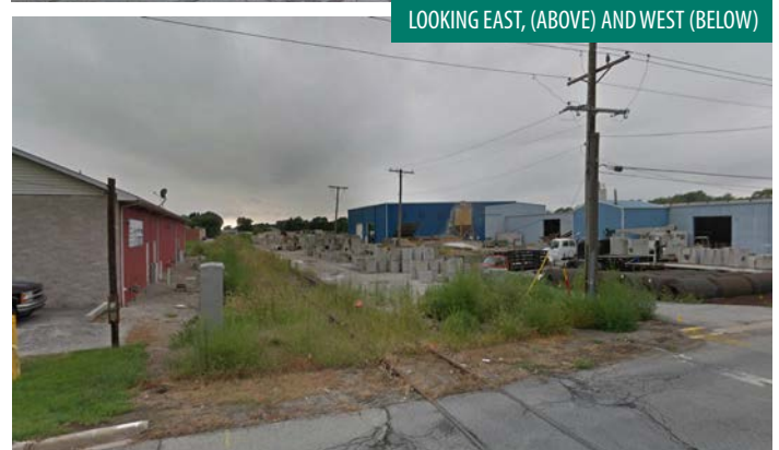
EXISTING RAIL R.O.W. LOOKING WEST FROM CALUMET AVENUE BRIDGE
